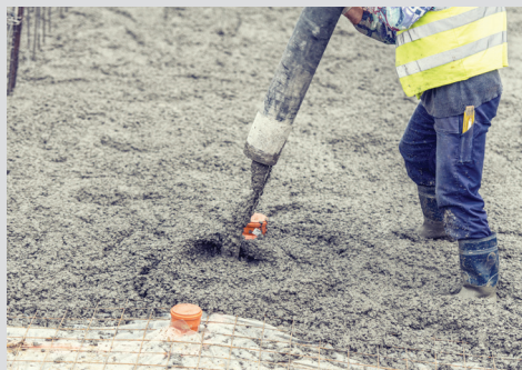
Transmitter starts measuring so you can start curing concrete
