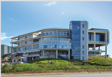
Tung Ho Steel Plant, Taiwan
