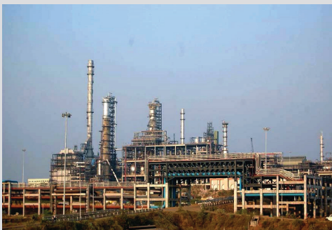
Bharat Oman Refinery, Bina, India
