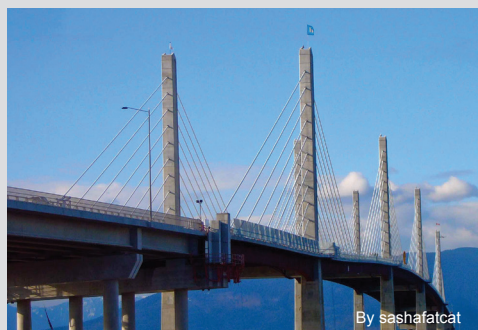
Golden Ears Bridge, Langley, Canada
