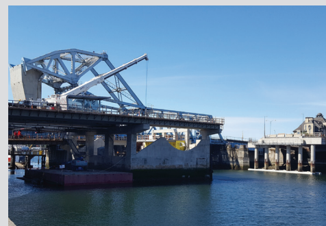
Johnson Street Bridge, Victoria, Canada
