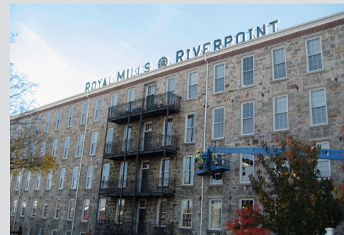
Royal Mills Apartments, Rhode Island, USA
