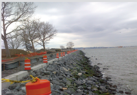
Governors Island Seawall, New York City, USA
