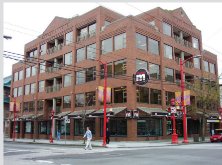
Channel M Building, Vancouver, Canada
